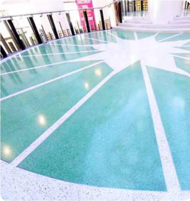
Harsh cleaning materials may cause damage to the terrazzo surface. All purpose cleaning products or those containing water-soluble, inorganic and crystallising salts, as well as harmful acids or alkalis should be avoided. Sealers recommended by the manufacturer can also be used to eliminate wear patterns caused by long periods of heavy traffic.
