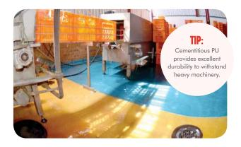
cleaning at 121°C should install a robust cementitious urethane screed, as they are much better in these situations than epoxy or methyl methacrylate floors. A system such as Flowfresh SR in a 9 mm thick layer will provide an effective barrier against the majority of extreme temperature situations encountered in a food and beverage facility.
