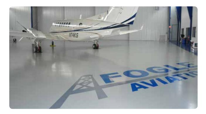
Anti-slip aggregates can be included within the resin make up of an epoxy system to provide extra grip underfoot. The anti-slip profile of the floor can even be tailored to meet the varying requirements of different areas of the hangar complex. This guide has been produced to give an overview of floor specification considerations when selecting suitable systems for use in aircraft hangars.
