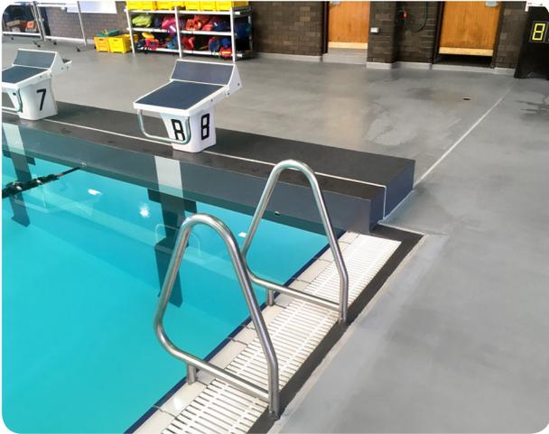
different cleaning and slip resistance priorities. By using epoxy systems, the specified coating doesn't need to change in different areas, just the amount of aggregate broadcast into the floor's resin matrix.
