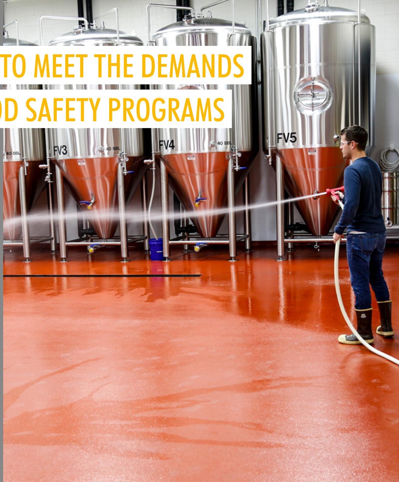
A rigorous cleaning process is essential to ensuring that contaminants are quickly and effectively removed – however the cleaning regime itself could pose a hazard unless the floor is durable enough to deal with it.
